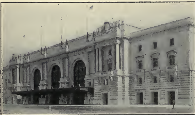
SAN FRANCISCO MUNICIPAL AUDITORIUM, WHERE THE CONVENTION IS TO BE HELD
